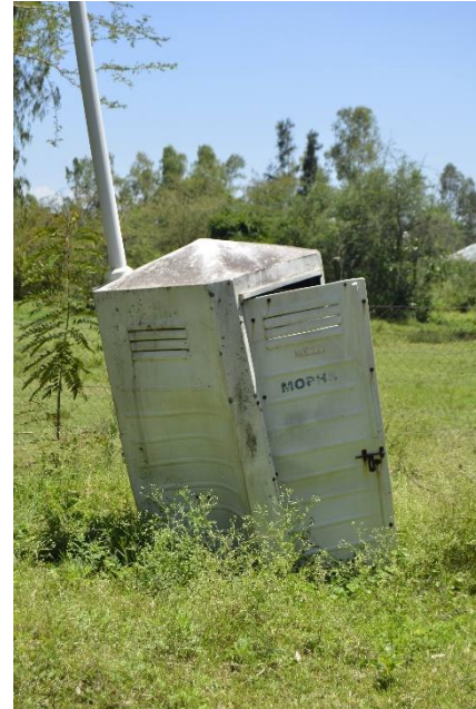
A community member demonstrating a collapsed toilet.
