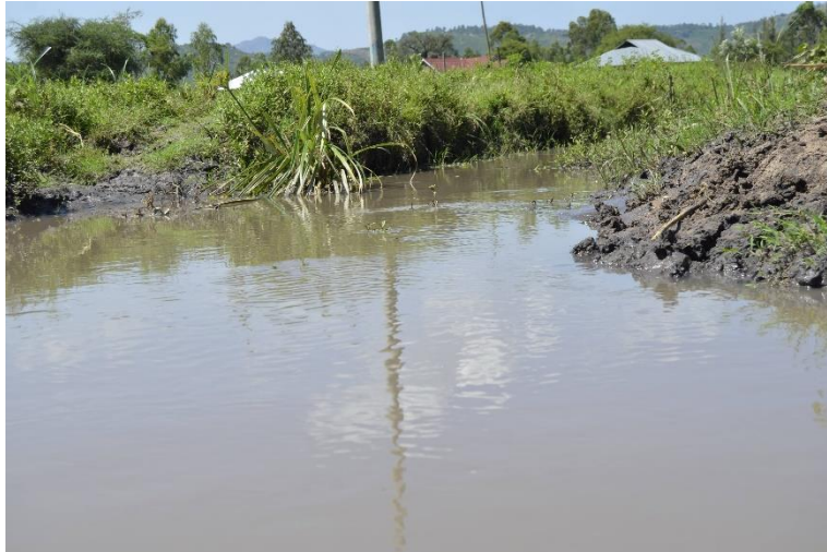
Flood water blocking the road.
