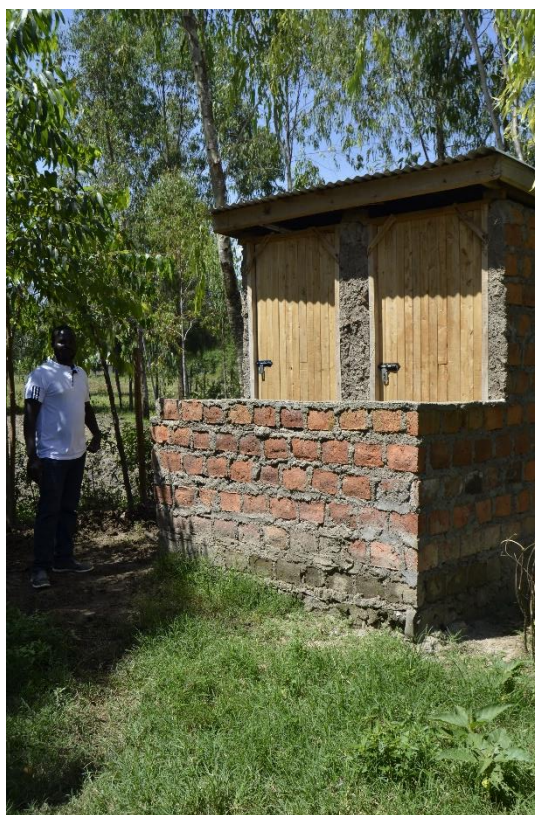
A recently constructed latrine
